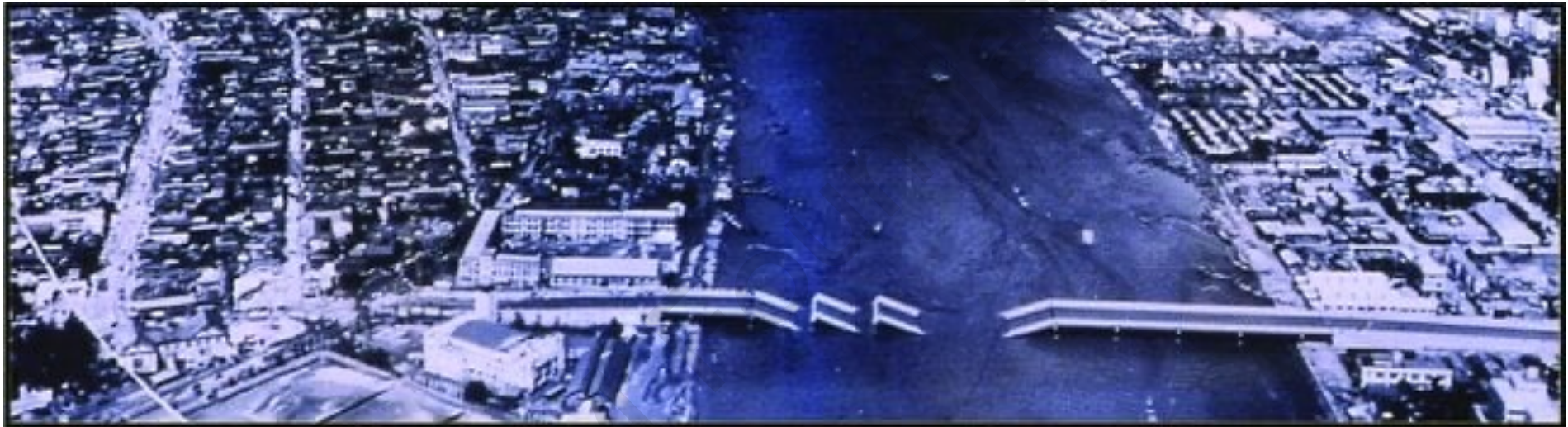
Collapse of the Showa bridge in Niigata, Japan
